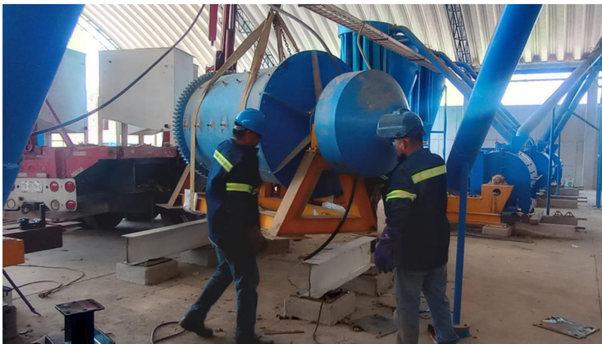
Figure 2 – Mounting of Ball Mill #1.
