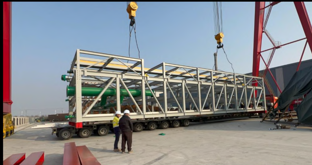
Pipe Rack Assembly
