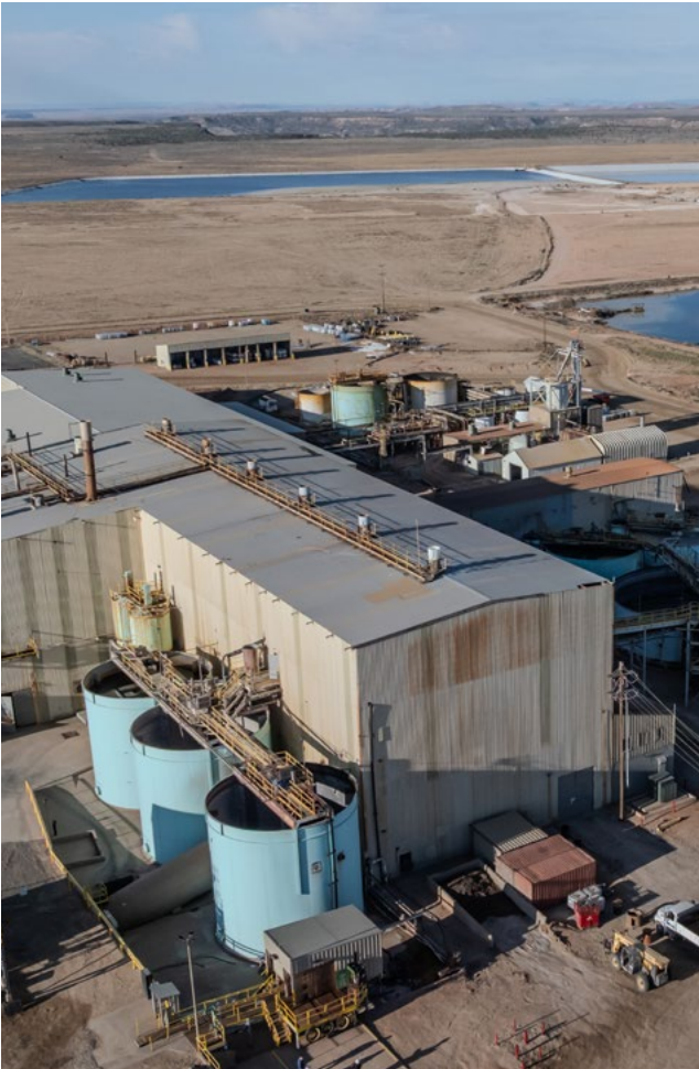
The White Mesa Mill manages uranium mill tailings and approved materials – including 11e.(2) byproduct material – in an engineered tailings storage facility designed for long-term containment and environmental protection.
