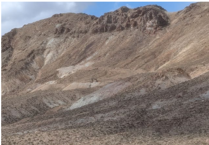
Figure 5: Drill Pad Construction at Sealy Ridge
