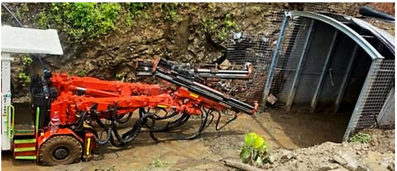
Figure 1 – Development jumbo entering new mine portal at Dittmer.
