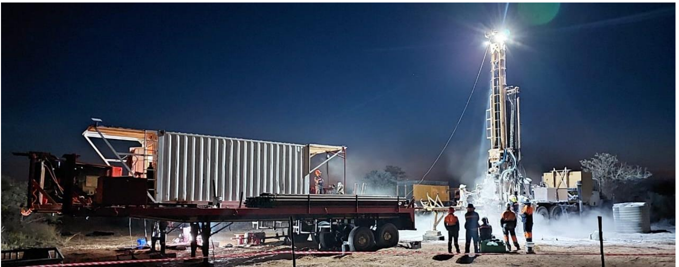
Figure 1. Well 3.5B spudding (Source: Botala)
