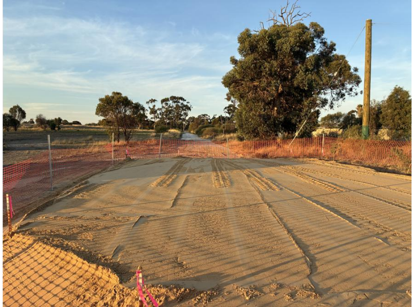
Site works for installation of electrical supply
