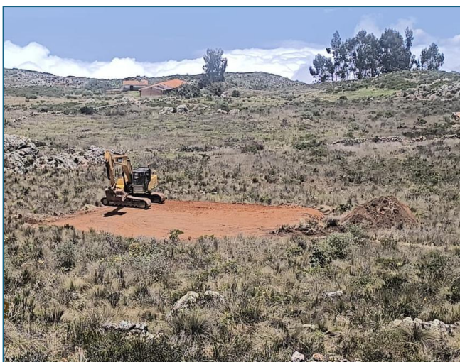
Image 3: Drill pads at Flint
