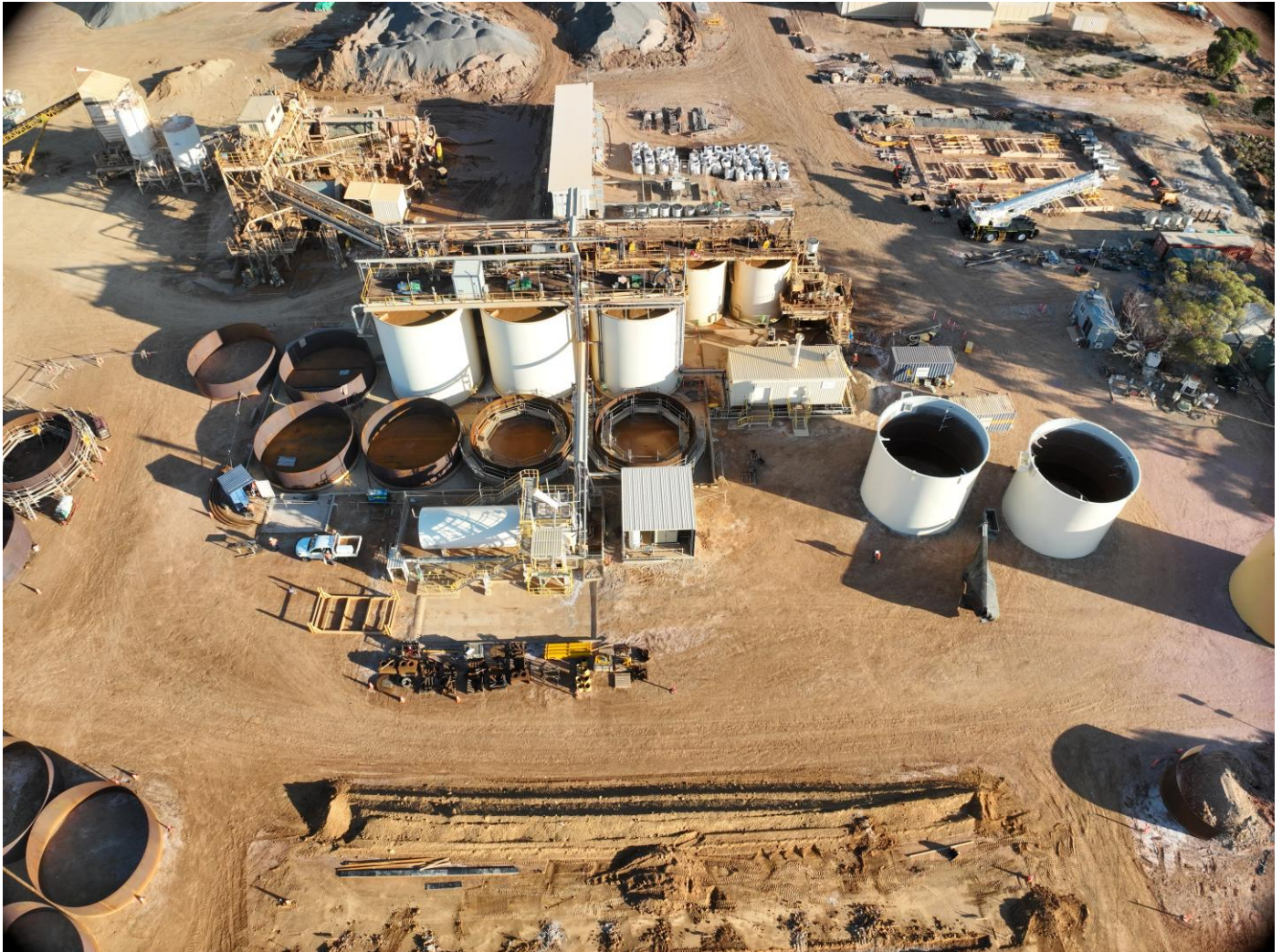
Image 3 – Jaurdi Gold Project Mill Upgrade – 28 April 2026
