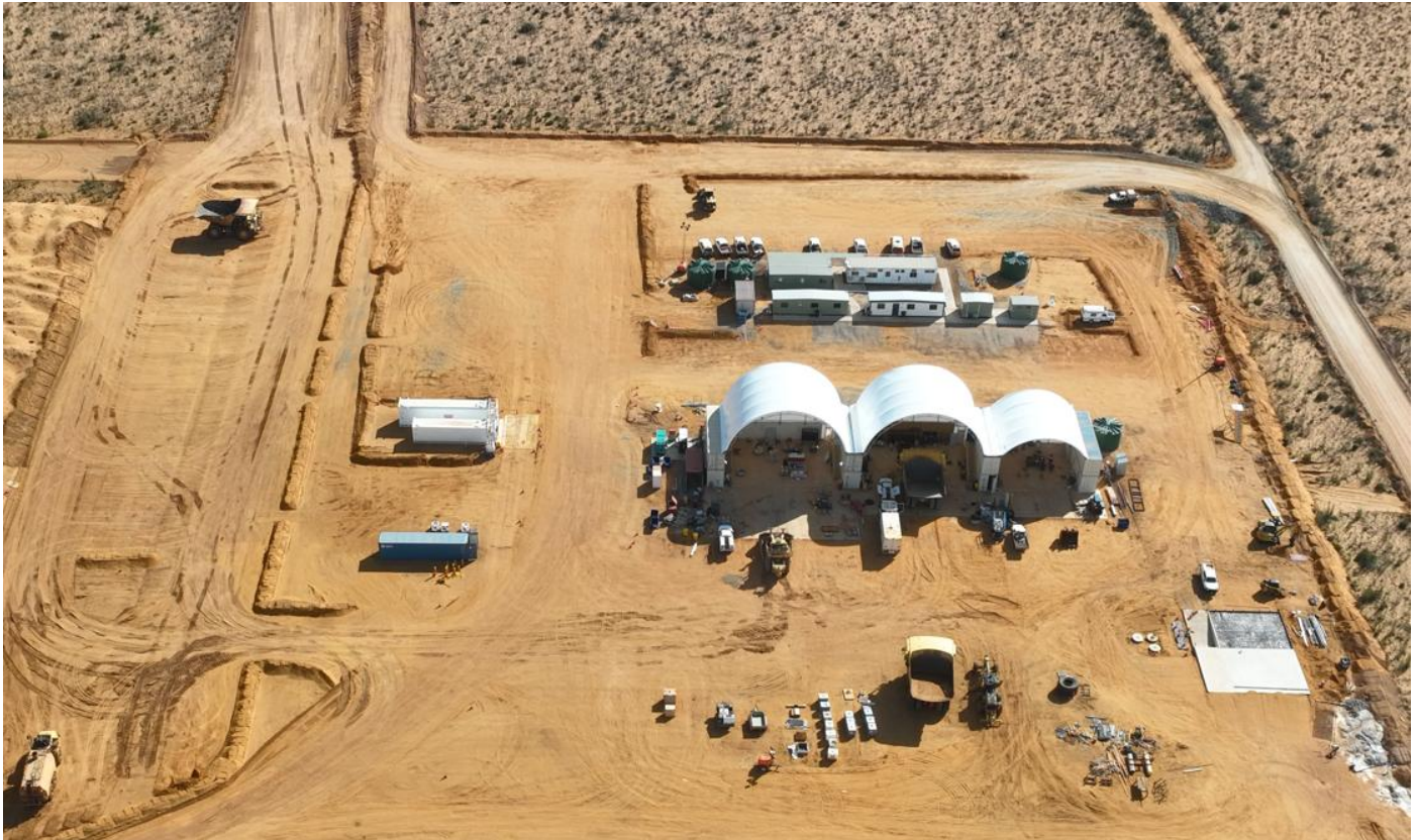
Image 2: Workshops and Infrastructure 20 April 2026
