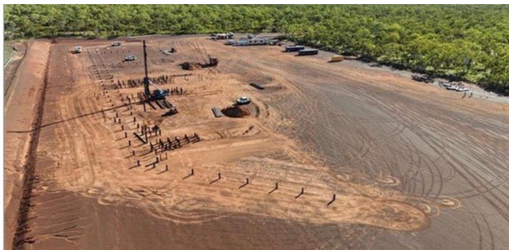
Civils and piling complete at the Carpentaria site in early April
