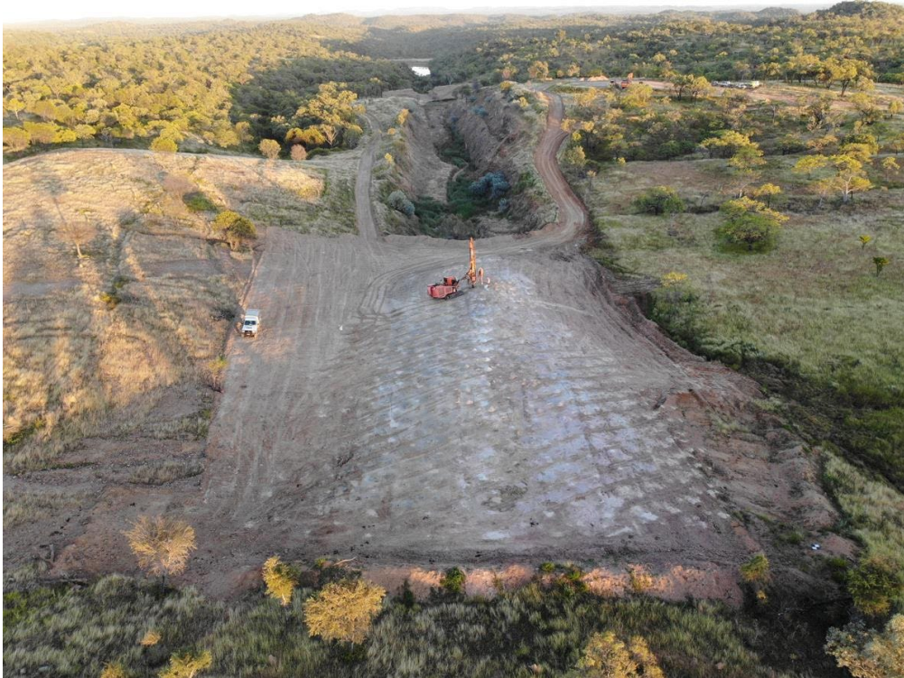
Figure 1: Drilling of first blast at Big Reef open pit
