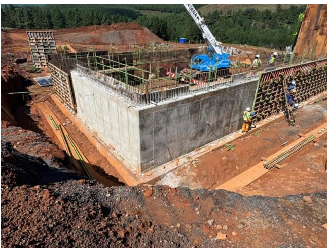
Figure 7: Gold Room Wall Progress – formwork removal
