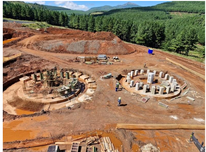
Figure 6 : Thickener Tank foundations in progress
