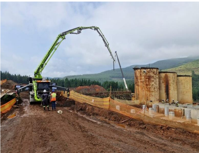
Figure 5: Concrete Pumping - Gold Room
