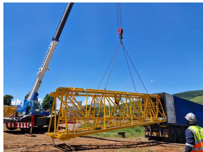
Figure 8: Tower Crane delivered to site
