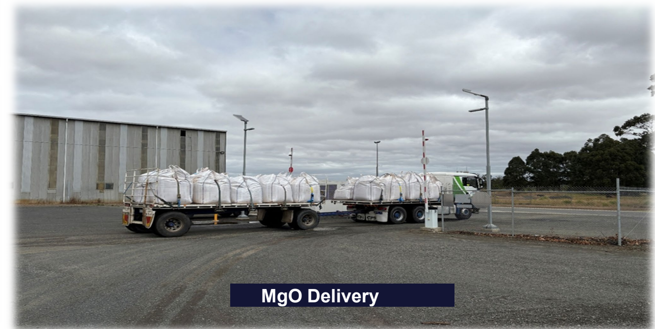
Reduction (Pyromet) Area Equipment – Pending Installation and Commissioning
