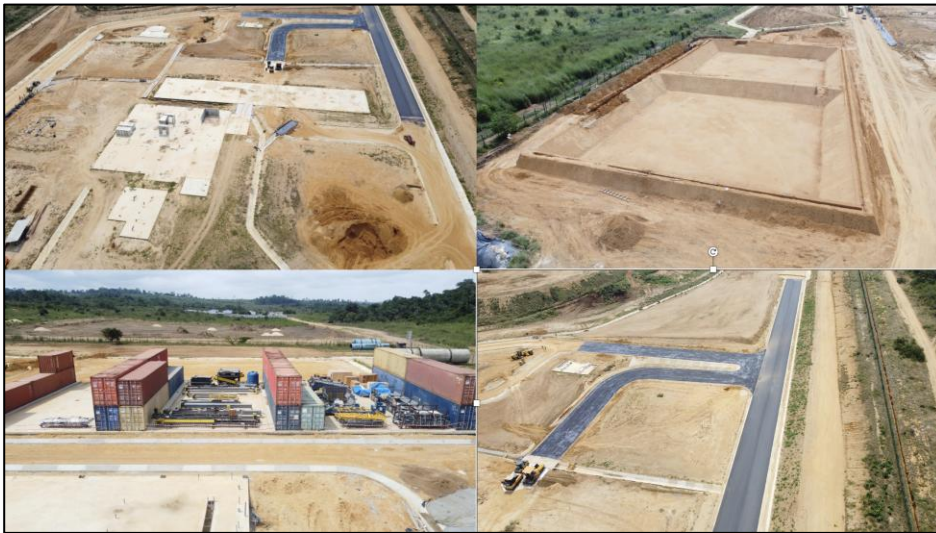
Figure 1 - progress at the Cabinda Phosphate fertilizer Project, located in Cabinda, Angola.
