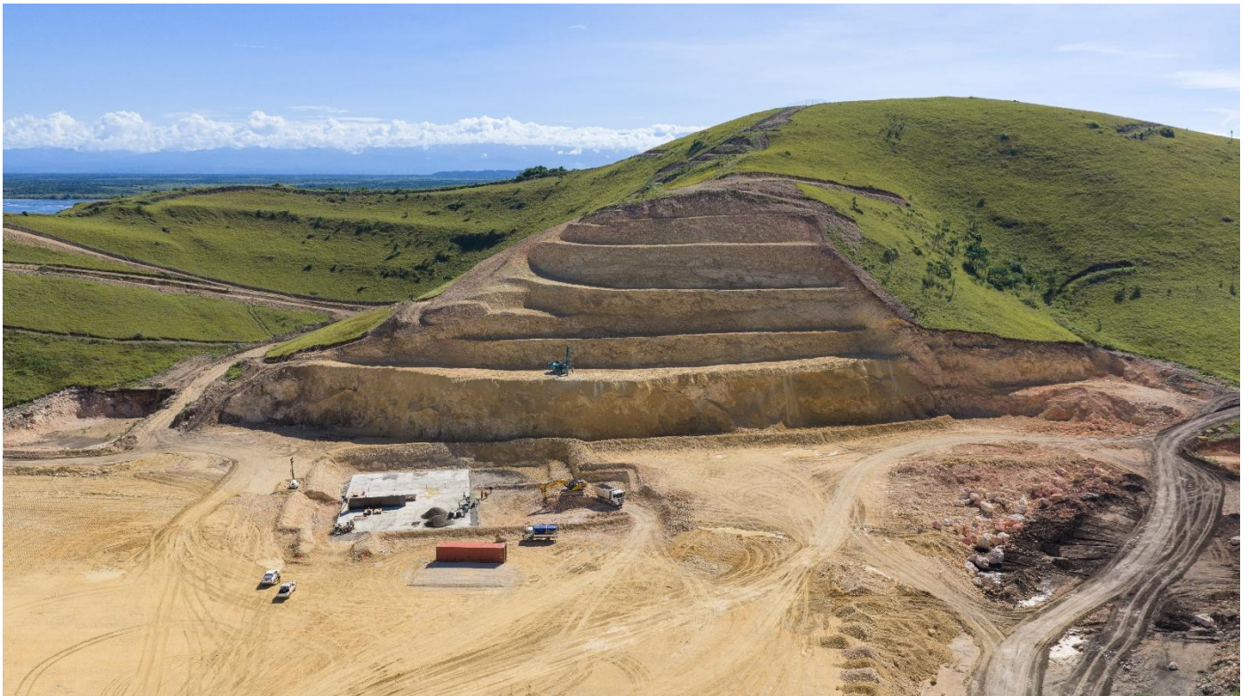
Image 2: Kiln pad areas trimmed and prepared.
