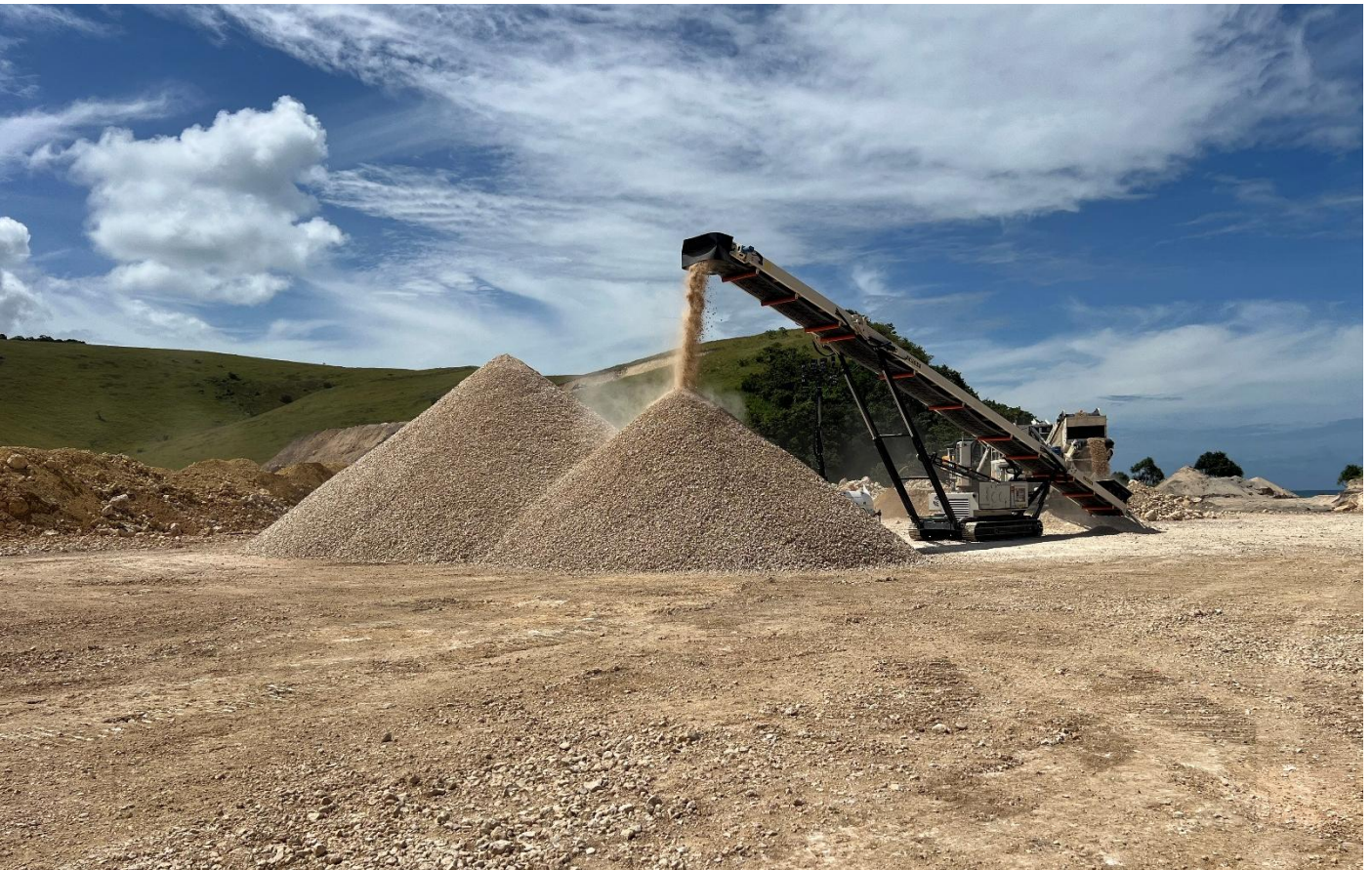
Image 8: Crushers have arrived on site.
