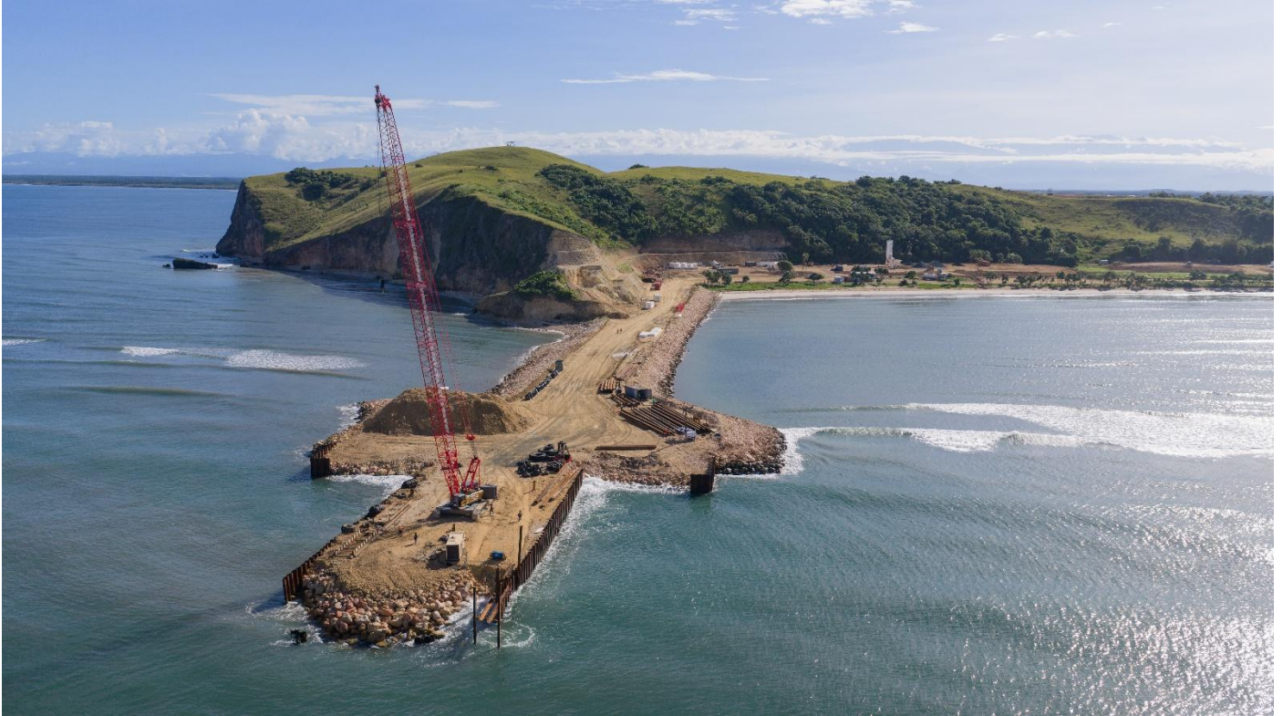
Image 1: Stage 3 of wharf construction underway.
