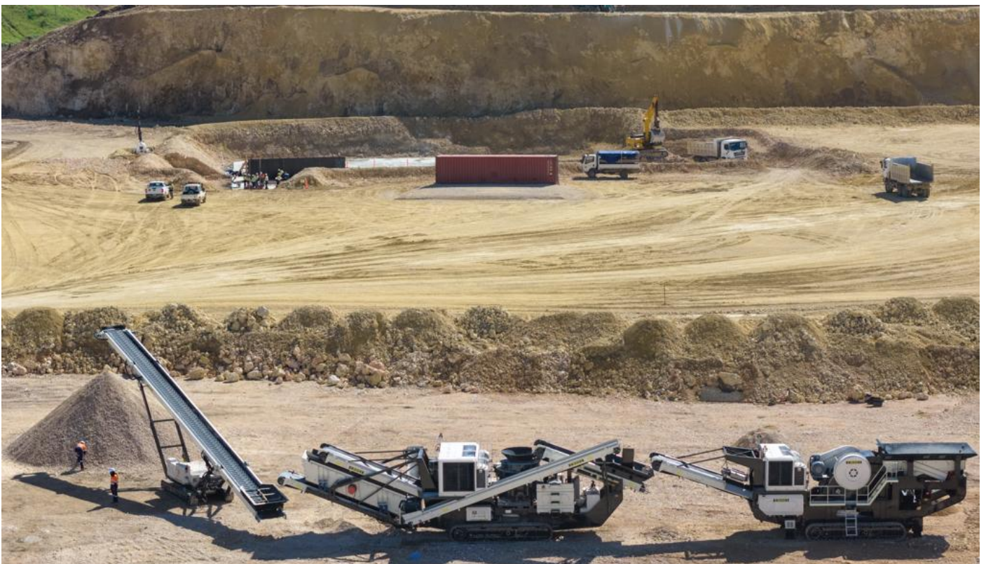
Crushers have arrived on site and commenced operation.
