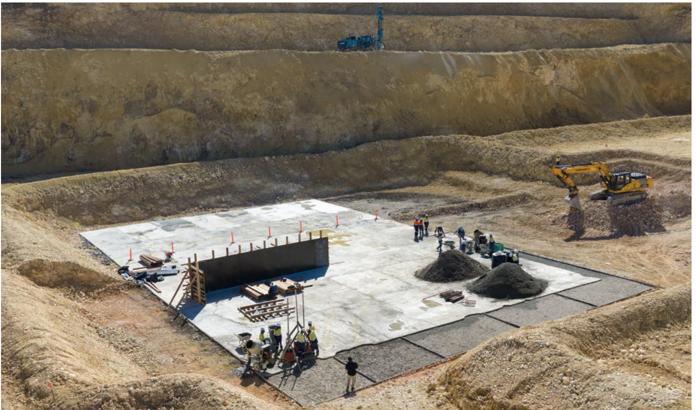
Kiln foundation works progressed through excavation with reinforcement and formwork commencing.
