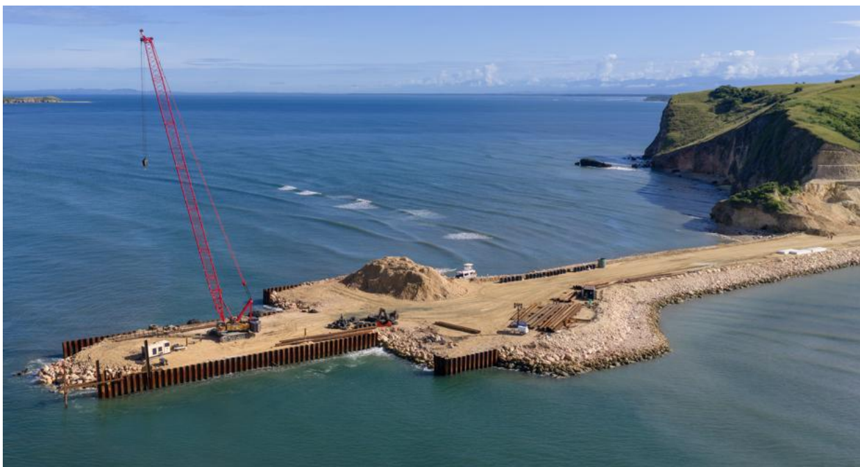
Stage 3 Construction of the Kido Wharf underway.
