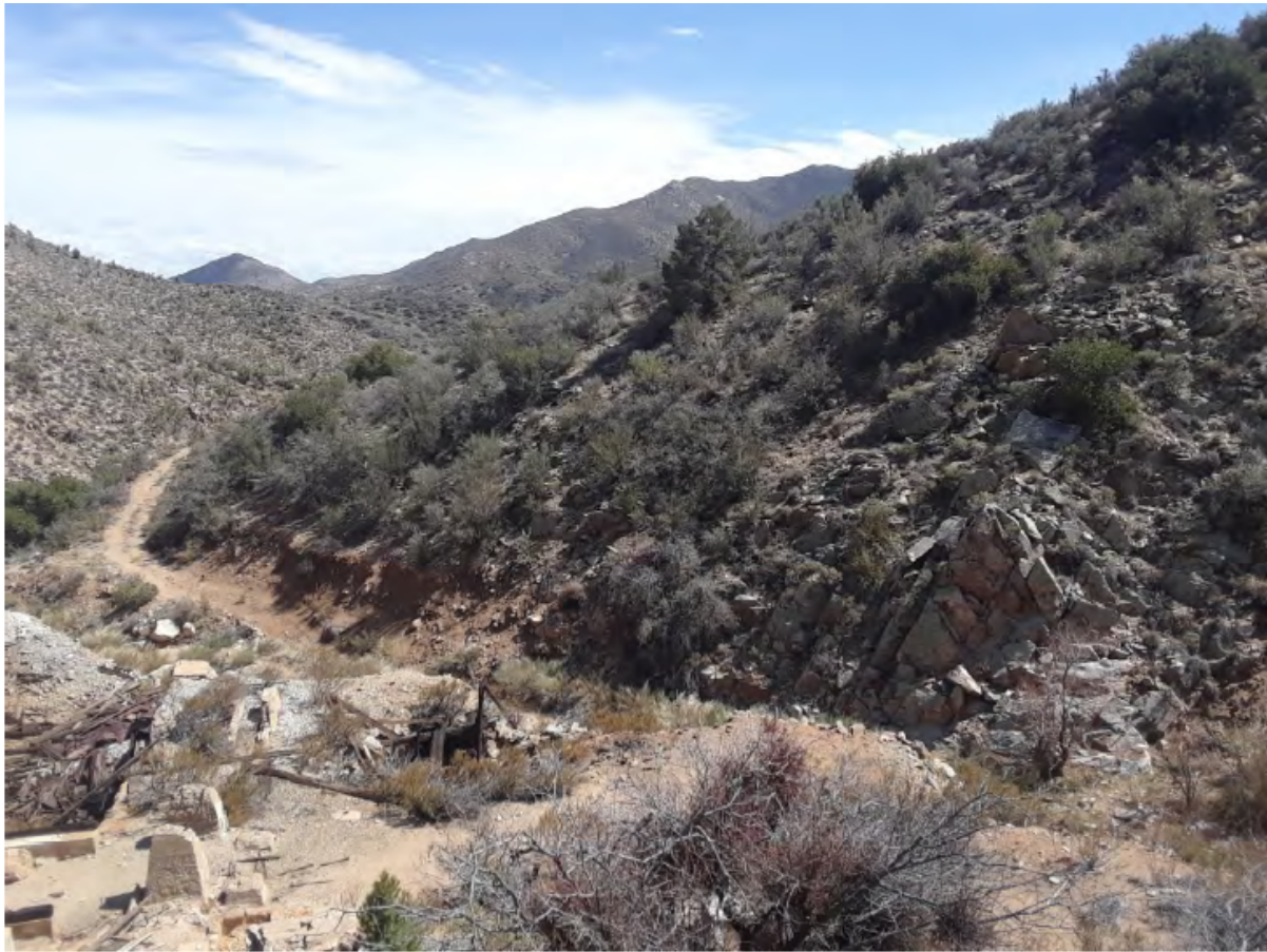
Figure 6: Residual surface infrastructure of historic Leviathan mine operations showing caved shaft (centre) and collapsed head frame and remnant foundations.
