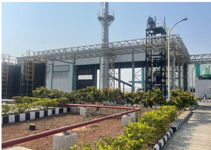
Figure 5: Part of the expanded Panthera Graphite Technologies facility.
