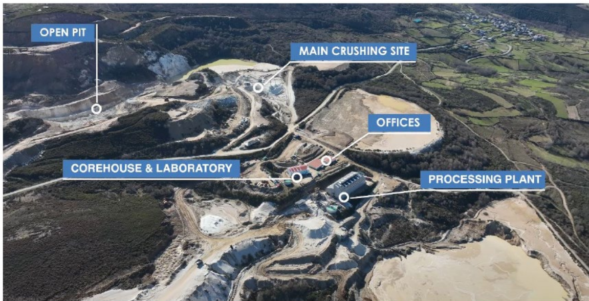
Figure 1: Overview of existing infrastructure at the Penouta mine
