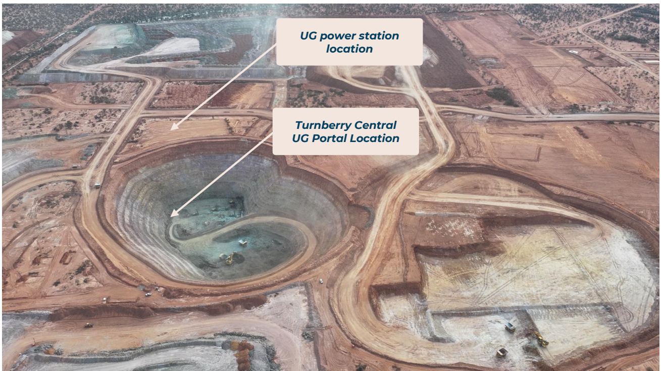
Figure 3: Turnberry Central (the location of the first underground portal) and waste stripping at Turnberry North, the final stage 1 oxide open pit to be mined (March 2026).
