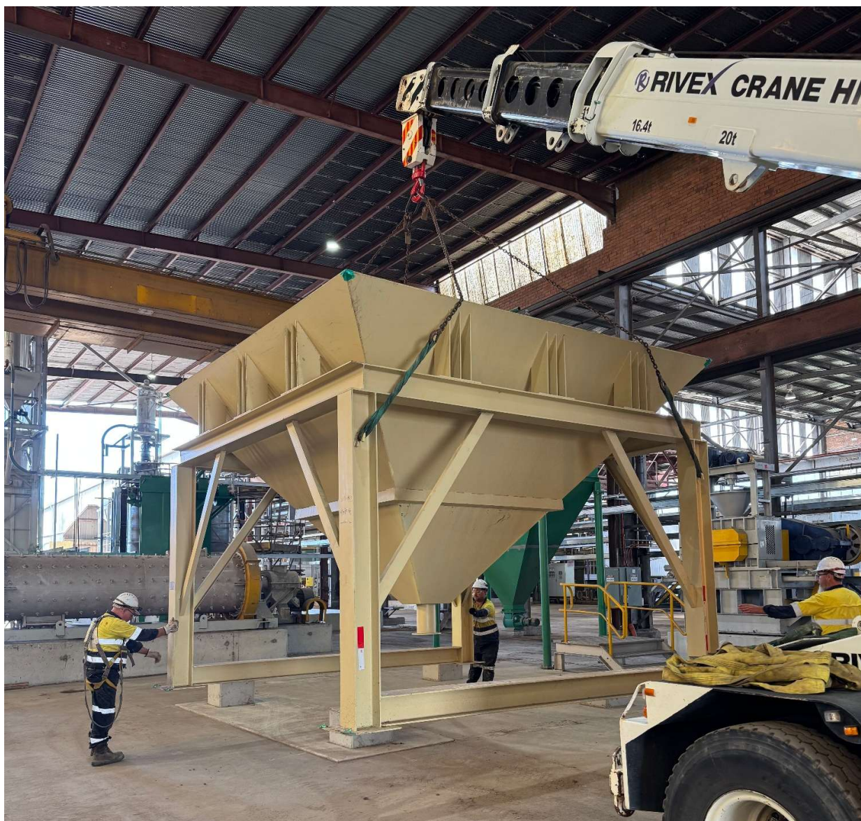
Heavy lift operations completed to position equipment (hopper) in their final installed location.
