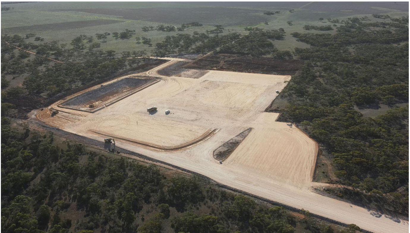
Processing Plant Pad Early Works Construction Completed
