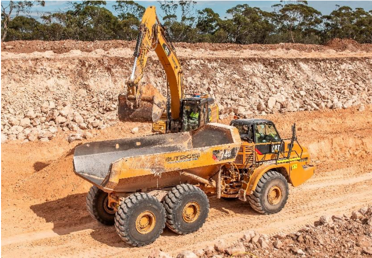
Excavation of the stormwater pond
