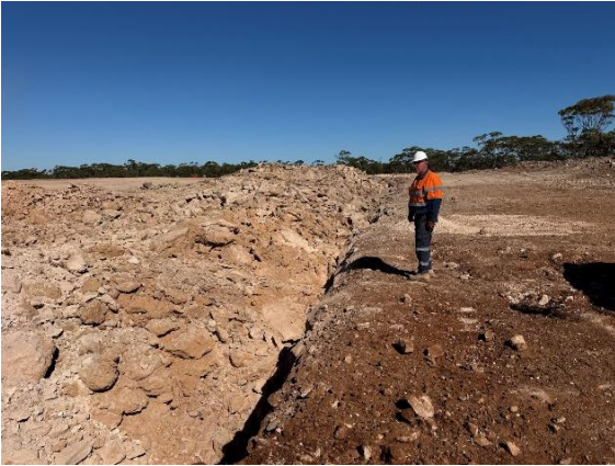
Post-blast inspection of the stormwater pond
