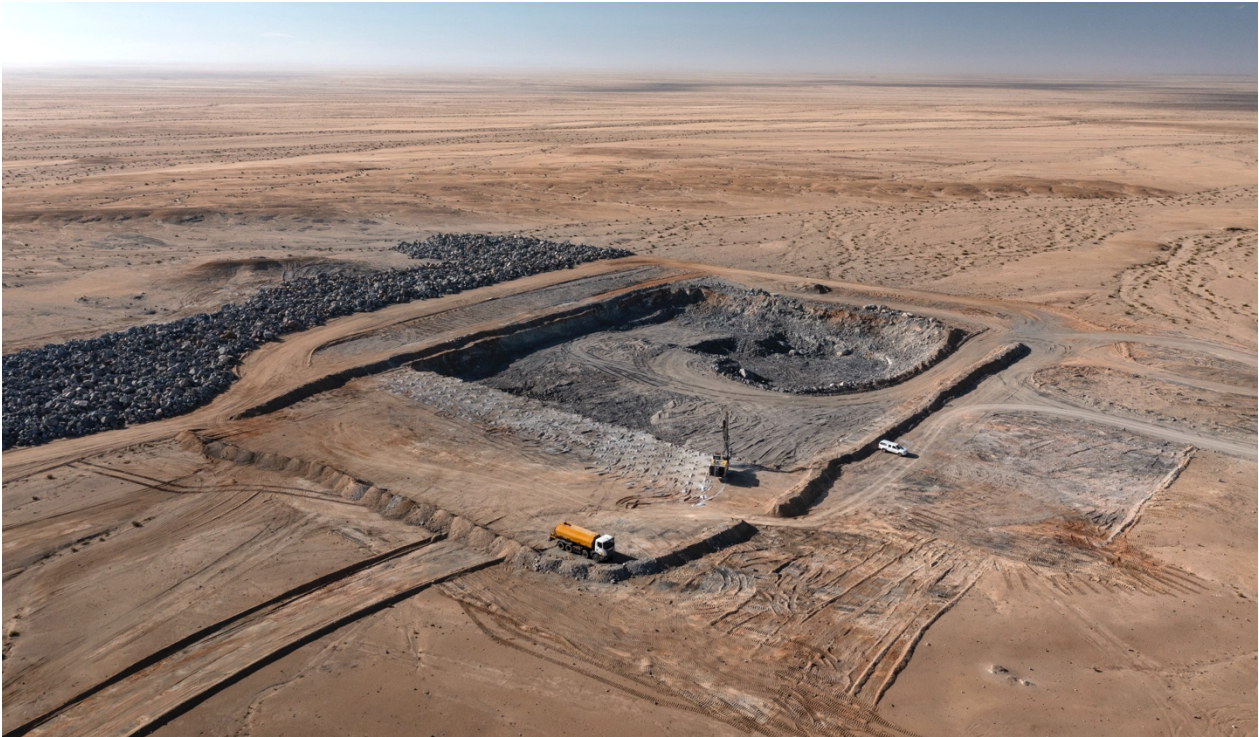
Figure 2: Blasting, crushing and screening of the heap leach drainage material.
