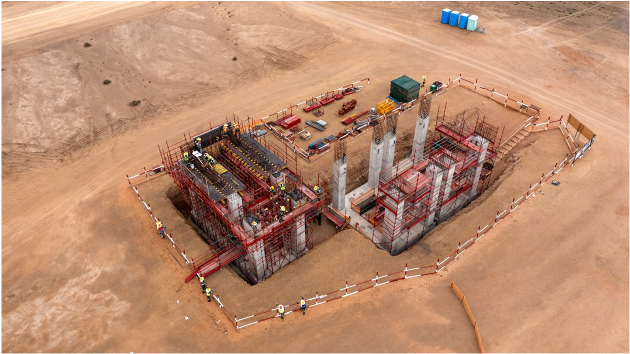
Figure 3: The base of the secondary and tertiary screening has been completed
