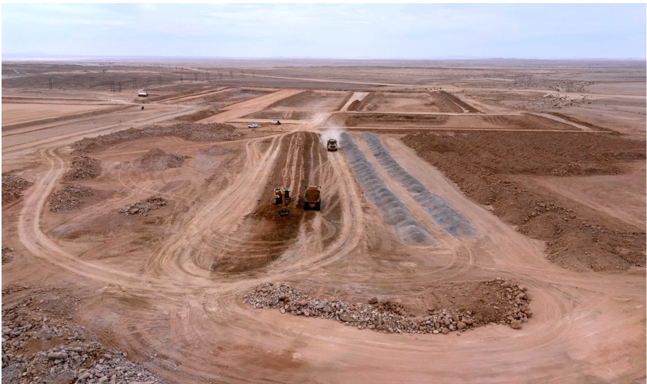
Figure 1: In addition to the heap leach pad earthworks, works have now begun on the wet plant terraces.
