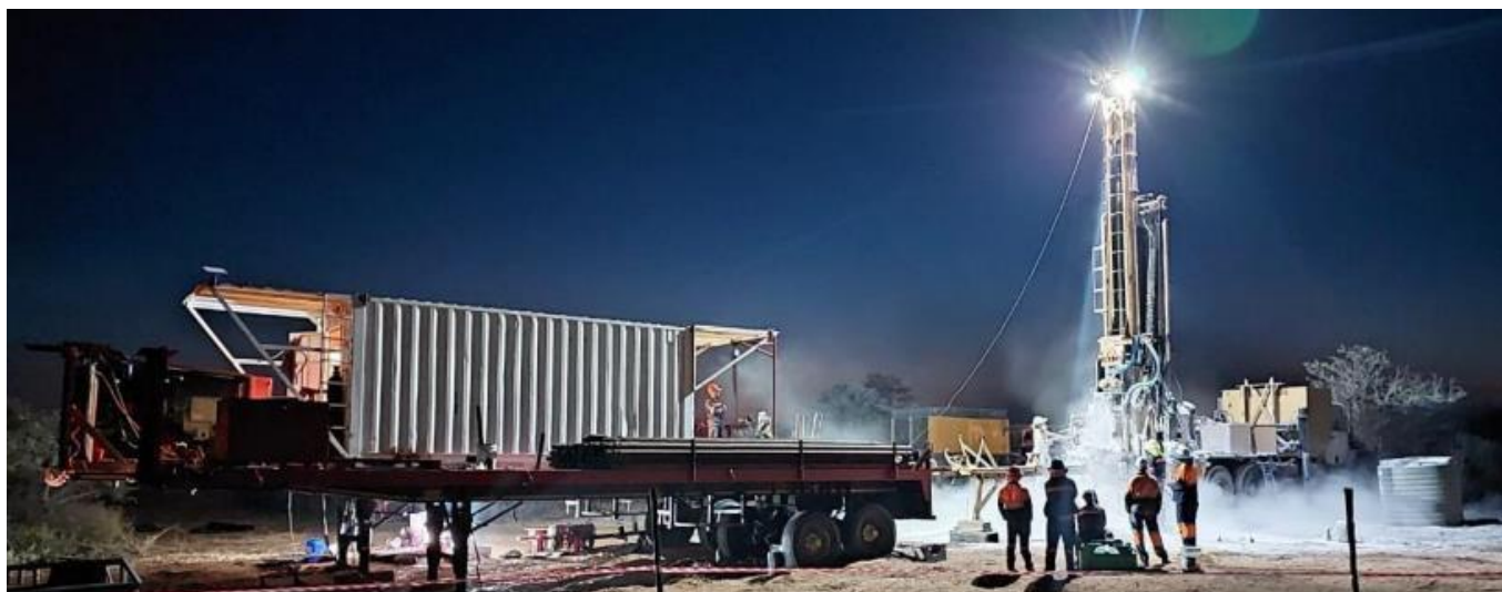
Figure 4. Pitse pilot well 3.5B spudding in late March.
