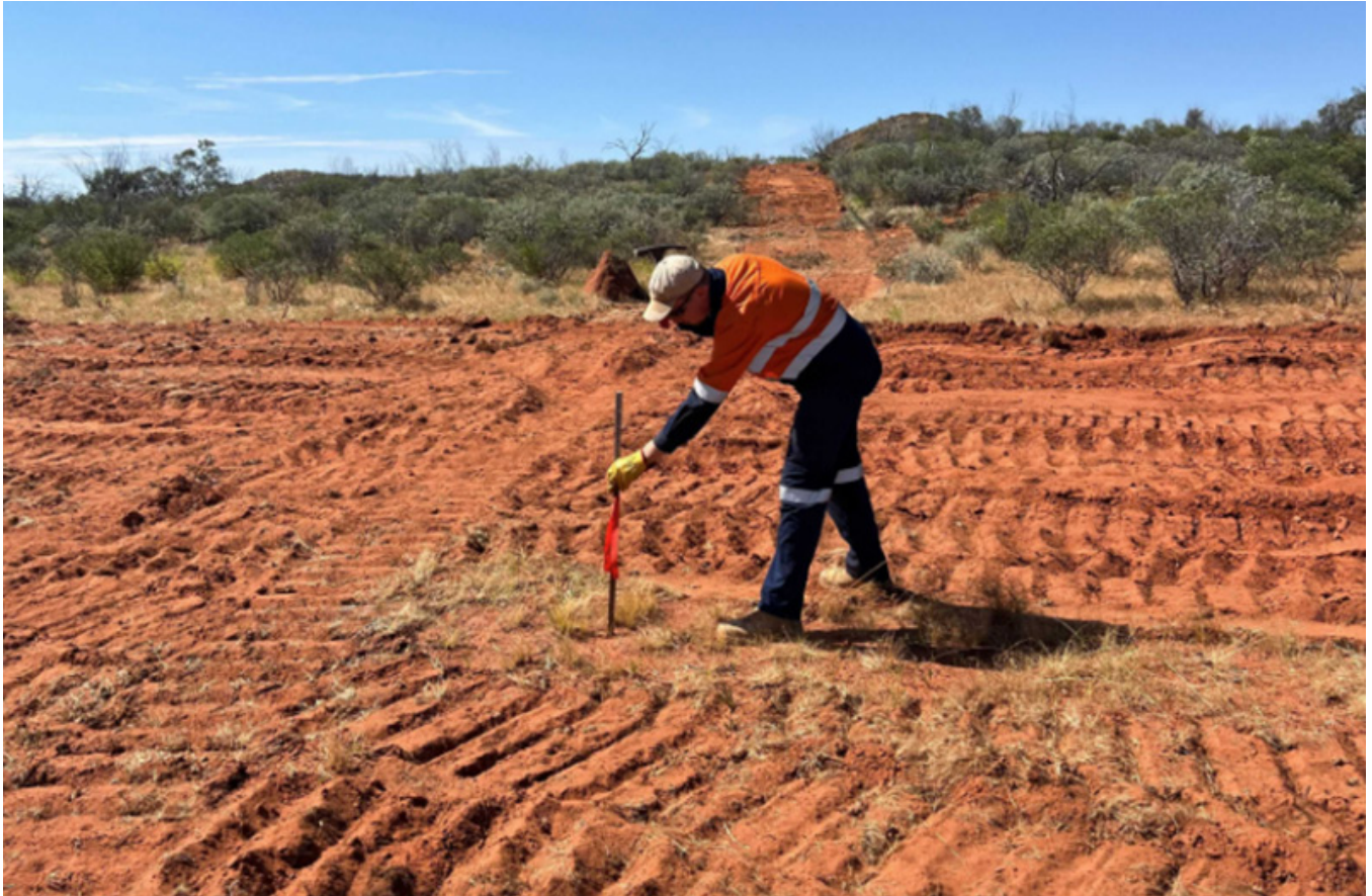
Figure 9: Pegging collar location for Stage One target at Molyhil
