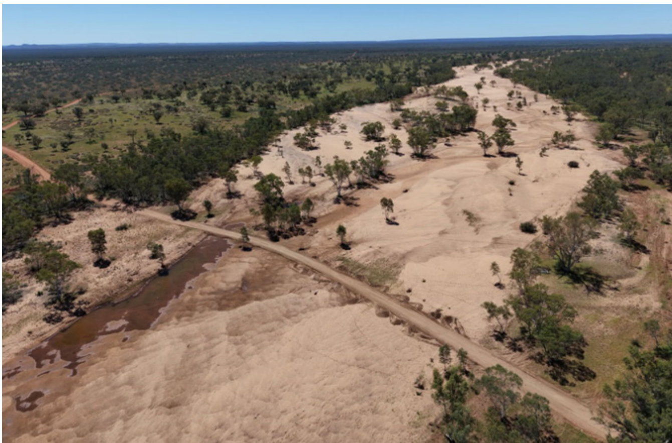
Figure 28: Photo of the existing Plenty River crossing track
