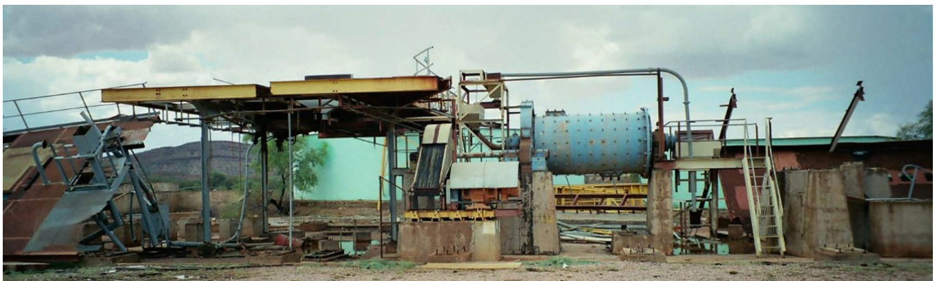
Figure 4: Historic Molyhil Process Plant Pre Site Rehabilitation (1998)
