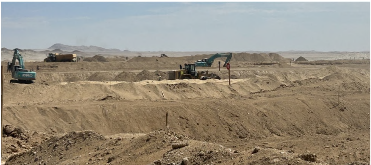
Figure 4: Bulk earthworks for the secondary mill area at the Tumas Project.
