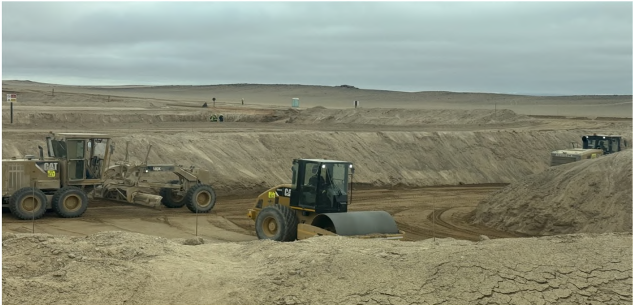
Figure 3: Bulk earthworks for the primary mill area at the Tumas Project.
