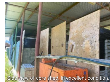
Side view of core shed. In excellent condition.
