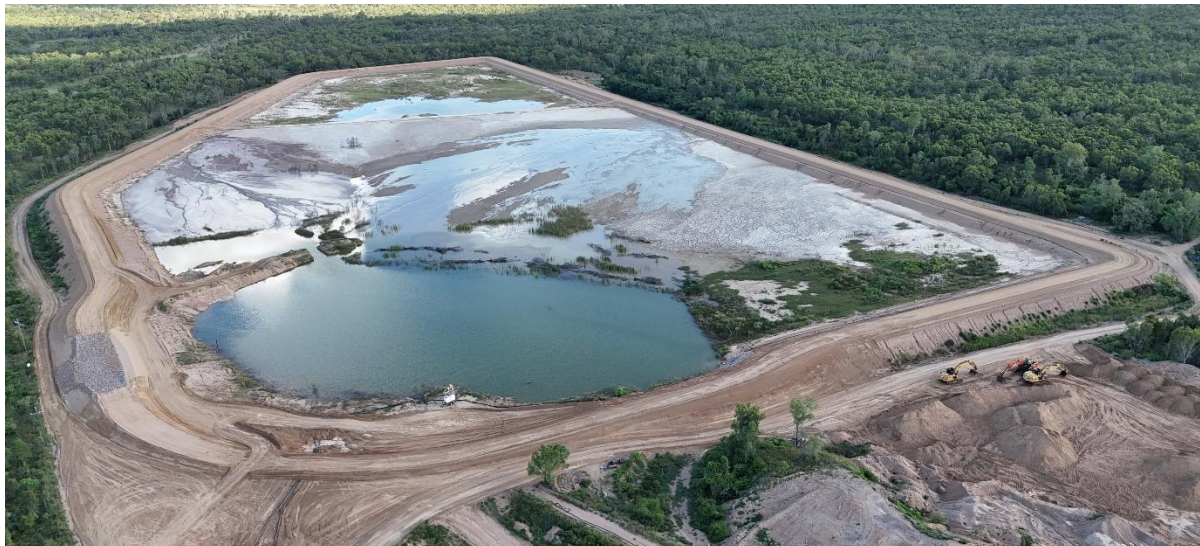
Figure 4: Overview of Blackjack TSF Stage 3 Lift Completed
