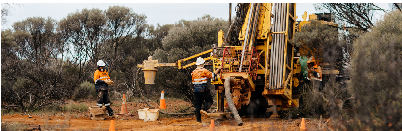
Figure 1. Drilling at Mt McKenna.
