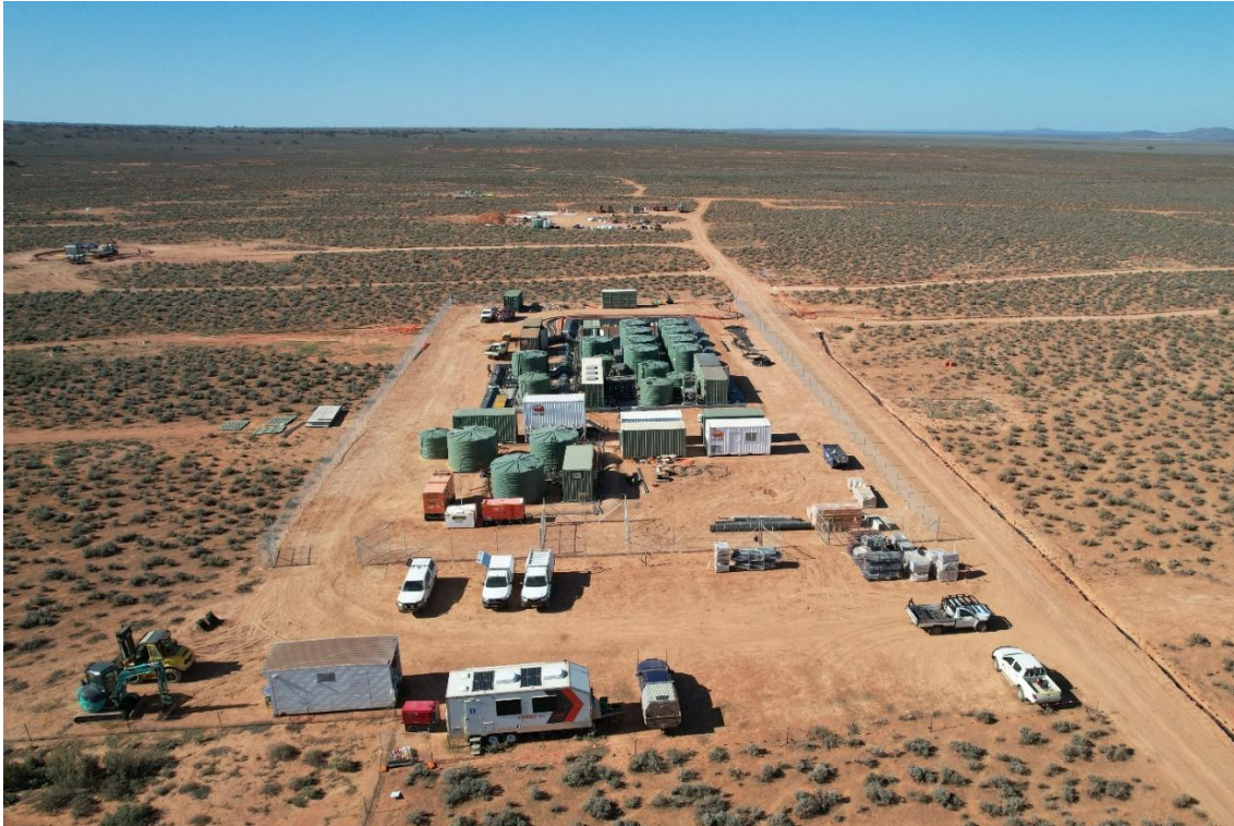
Figure 1: Samphire Field Recovery Trial Plant in full operation (view looking north)
