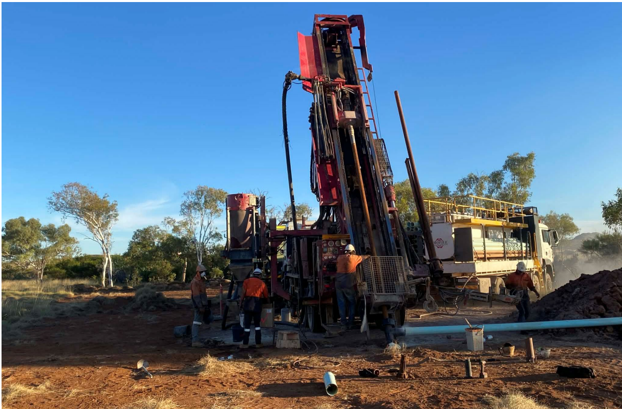
Figure 1: Profile Drilling Services RC Drill rig collaring the first drillhole at Twin Veins Prospect, Marble Bar Gold Project.
