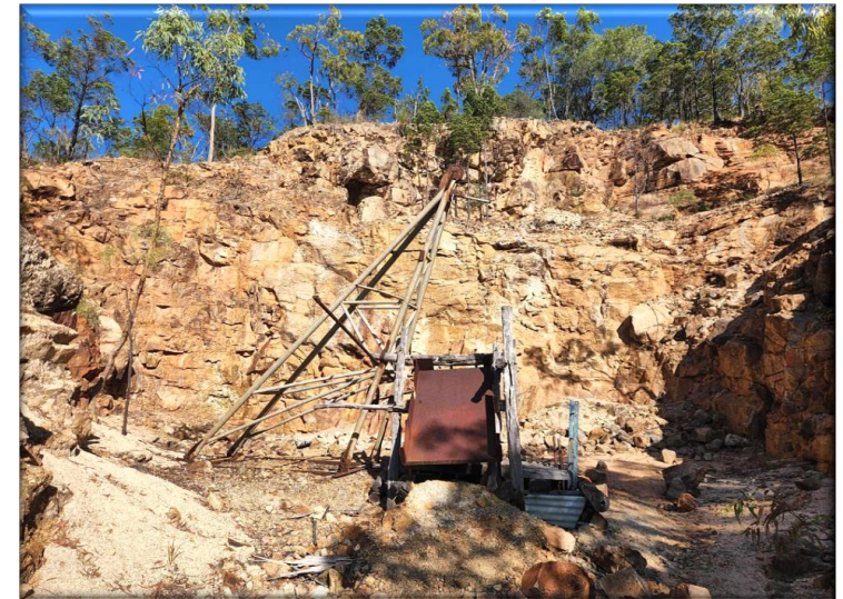
Daisy Bell open cut with exploratory shaft headframe still intact
