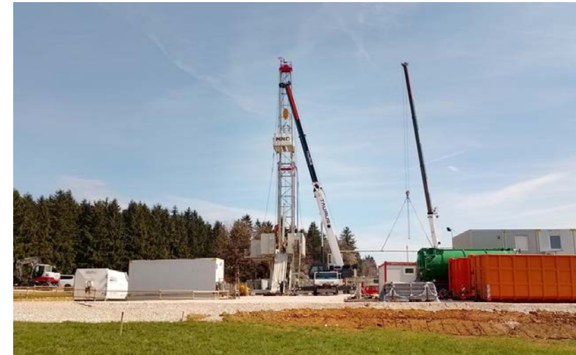
Rig up at the HOCH-1 drilling location
