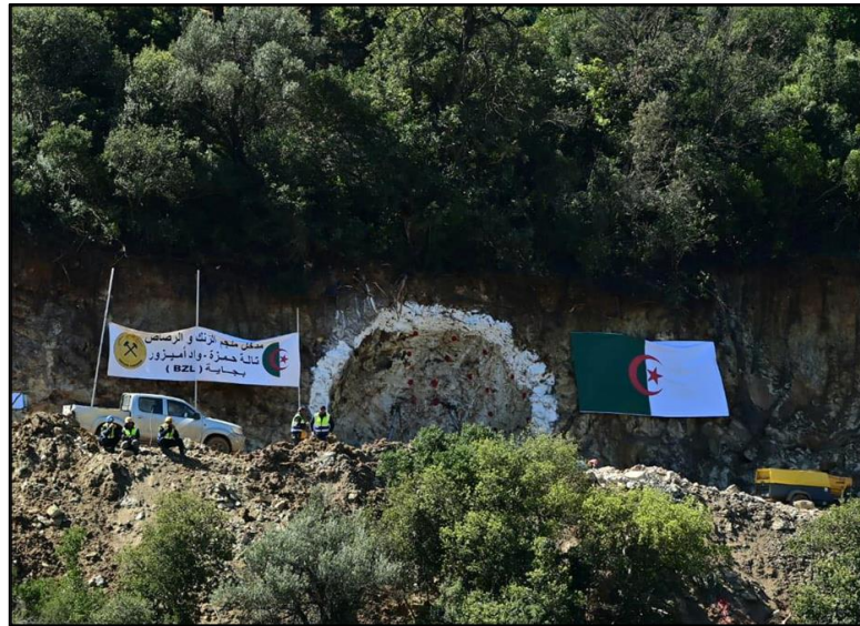
Figure 2: Early access works at the site of the portal
