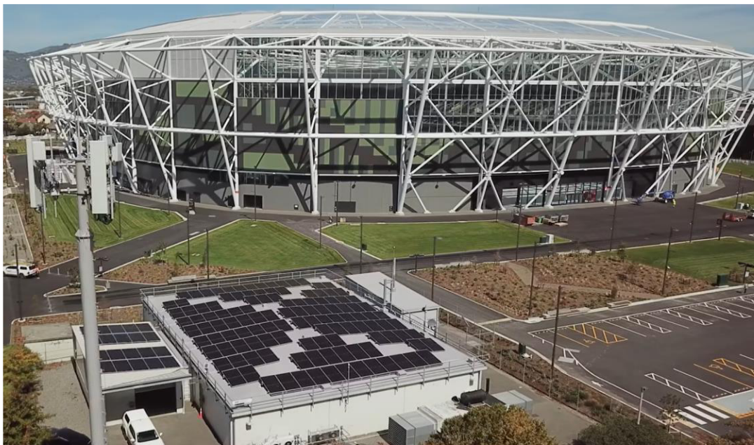
The data centre and mobile tower (foreground) adjacent to the new stadium.
