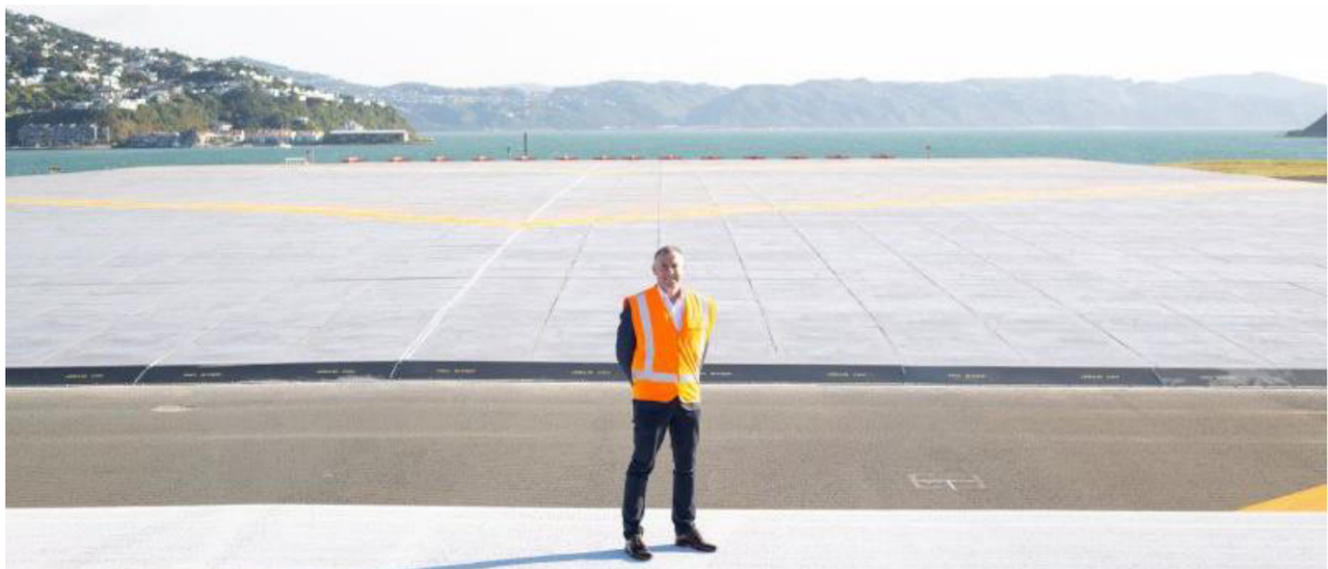
Wellington Airport CEO Matt Clarke in front of the completed northern safety area.
