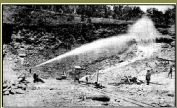
High pressure sluice mining used at the Mount Sheba Mine, Nundle Gold Field, 1890's.
