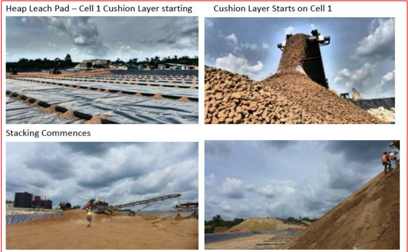
Figure 4: Heap Leach Pad and Pond Section
