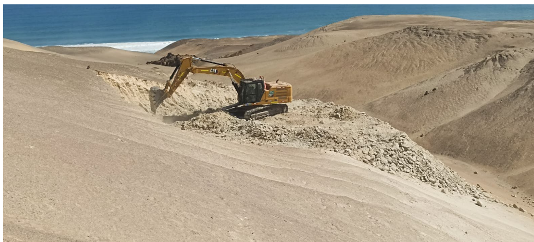
Figure 5: Playa Kali IOCG Project showing drill pad preparations
