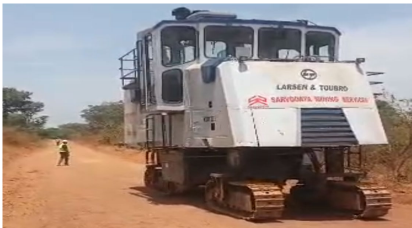
Image 3 and 4: Surface Miner Arriving on Site
