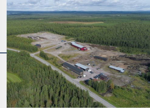
Existing KSB Project office and laydown area
