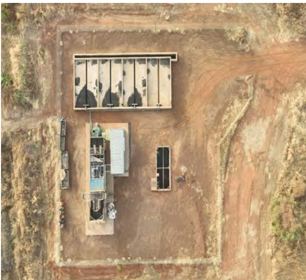
Kiaka wastewater treatment plant
