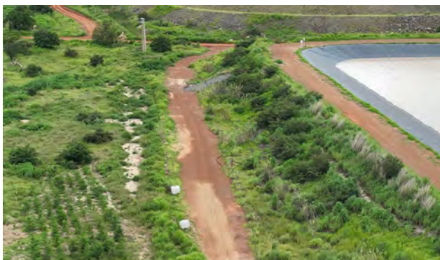
Progressive rehabilitation around Water Storage Facility, Sanbrado
