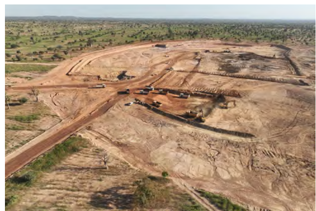
Preparatory works for Toega open pit
