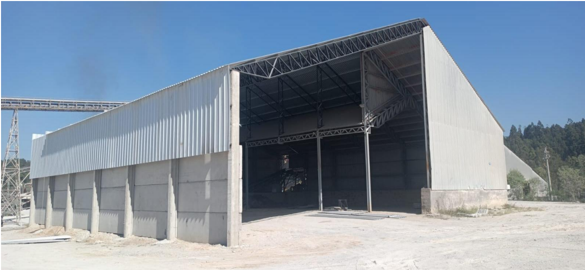
Photo 1 Run of Mine Storage complete
