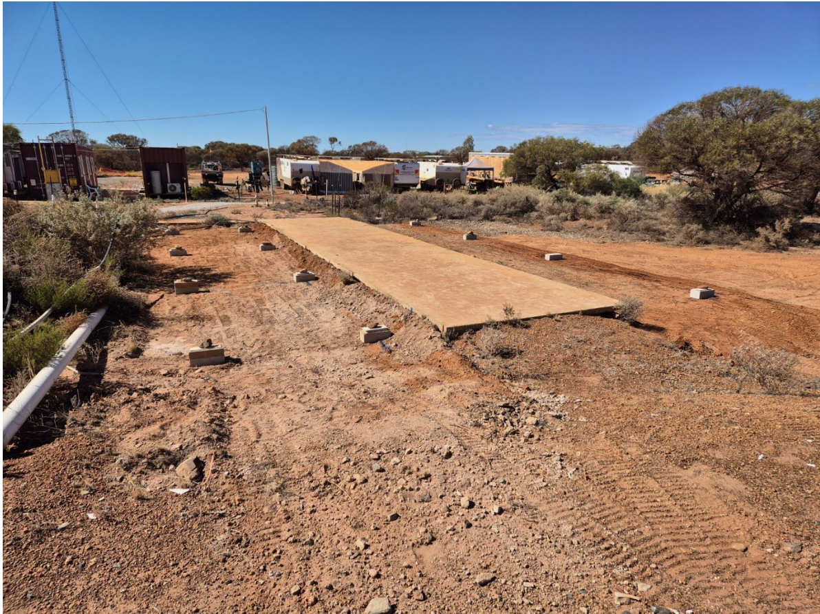
Figure 5 - Site preparation for additional accommodation units
