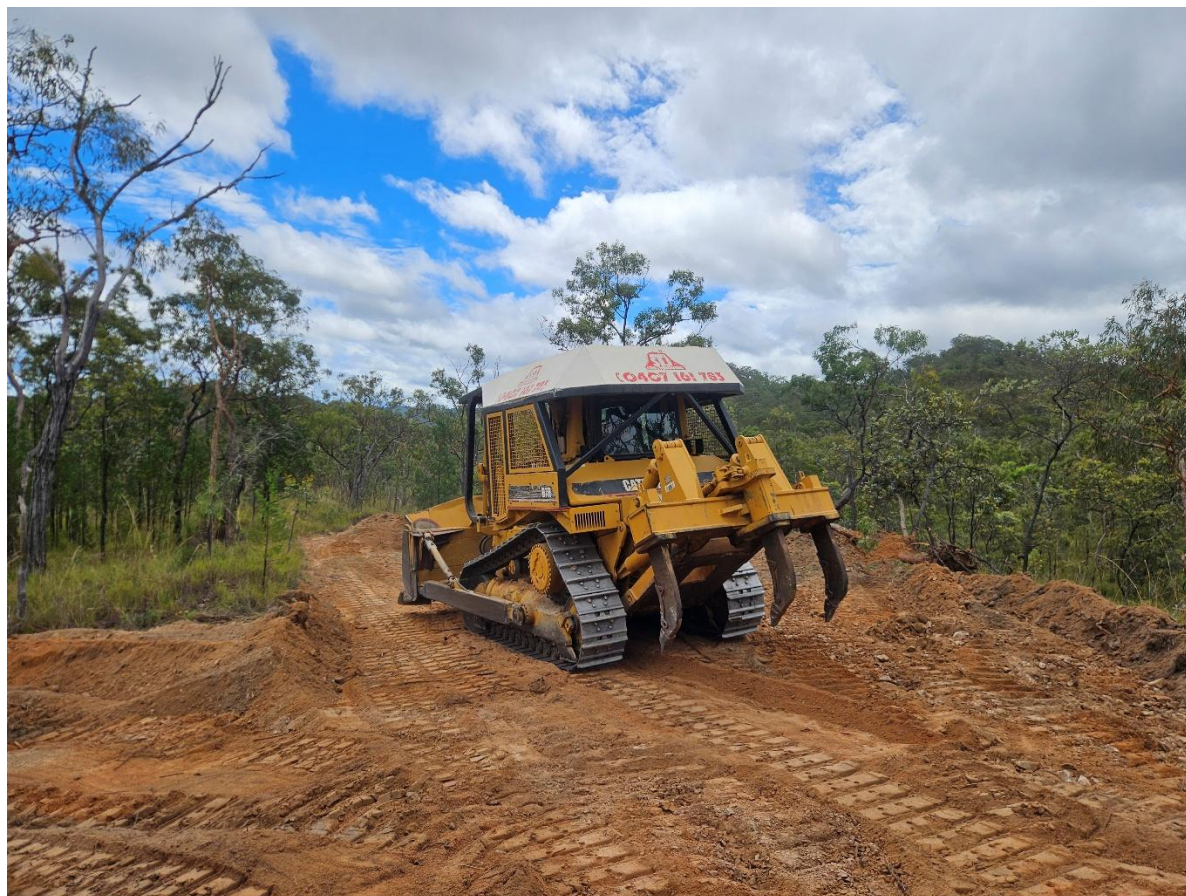
Figure 1 Bulldozer completing earthworks for drilling at Orient Project, Qld
