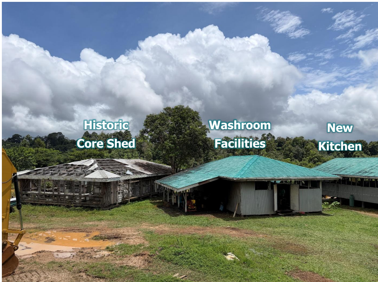
Figure 5: Location of North Peters camp buildings adjacent to historic core shed. View looking out of the office unit.
