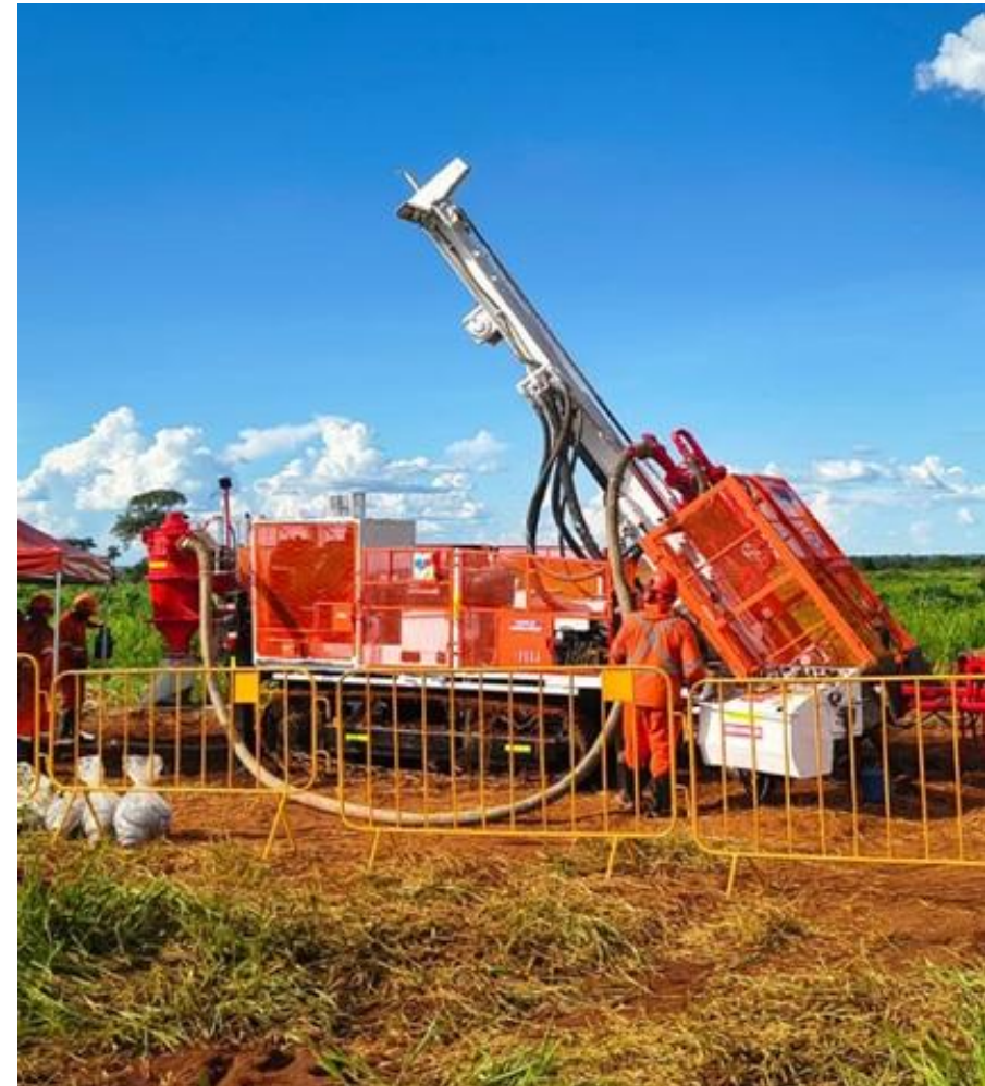
Drill rig on site at Santa Anna.
