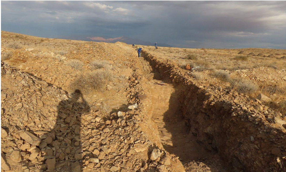
Image 1: Example of the trenching completed at the OP Target. Trenches are dug using a mechanised excavator to the point of refusal. The trenches are then cleaned manually and mapped by a geologist to document the exposed geology across the width of the pegmatite target and document the host lithology. Visual indicator marks are made across the pegmatite for channel sampling to be completed using a rock saw and hand chisel to remove the sample for bagging and sample preparation.
