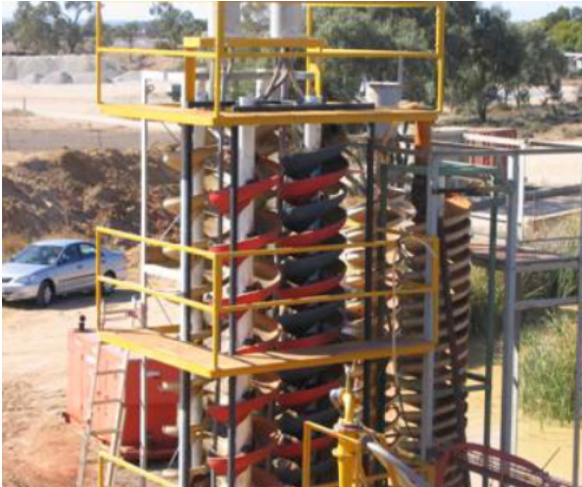
Figure 10-1: Donald historical wet concentrator pilot plant in 2005
