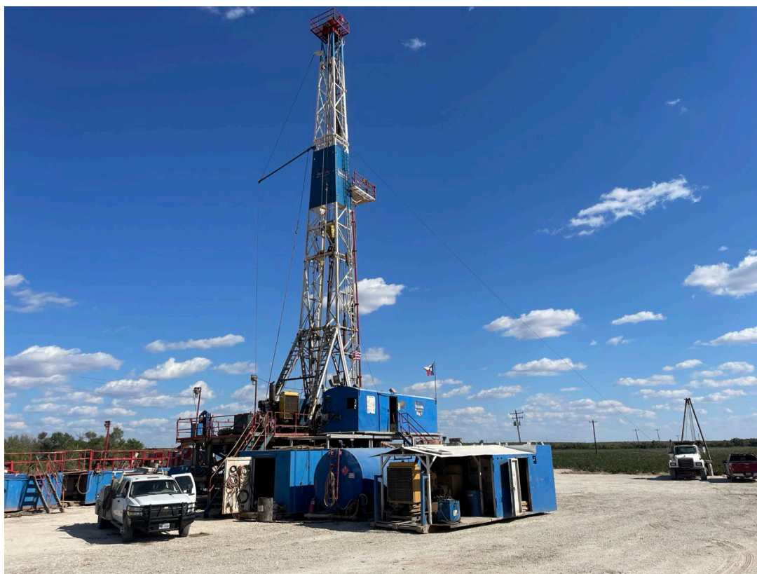
Photo 1: JVU-5 drilling operations at the Varn Oil Field
