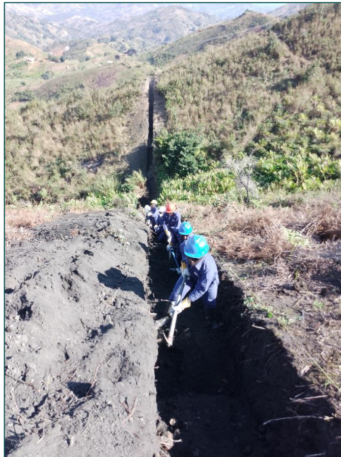
Photo 1: Excavation of trench TRUM23-002
