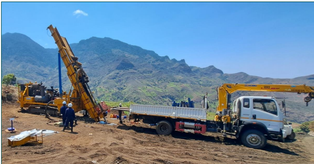
Photo 2: RC drill rig in operation at Kumba Deposit, Morogoro Graphite project, Tanzania.
